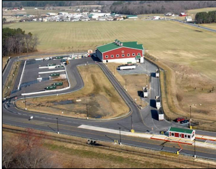
Plate 3-2: Sample waste transfer station
