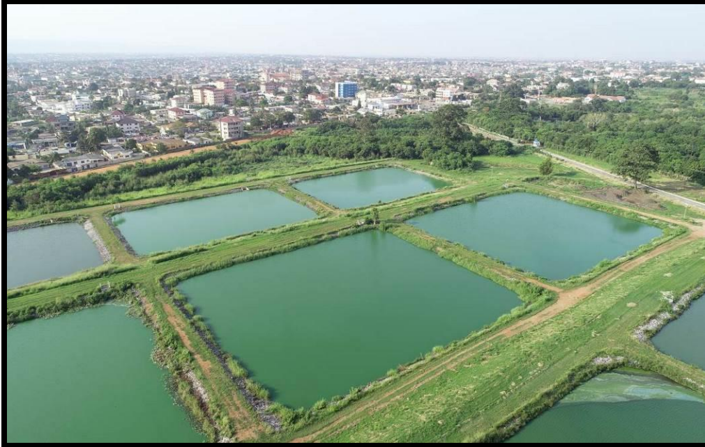
Plate 3-1: Sewage treatment ponds close to the proposed project site
