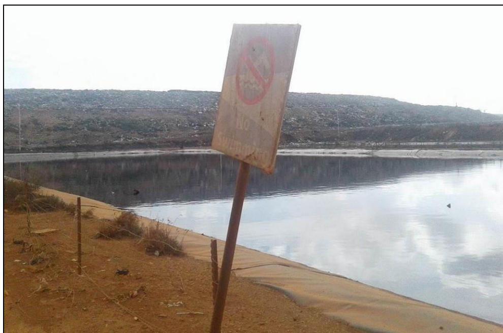
Plate 5-6: Fencing and warning sign by leachate pond, with dump site in the background
